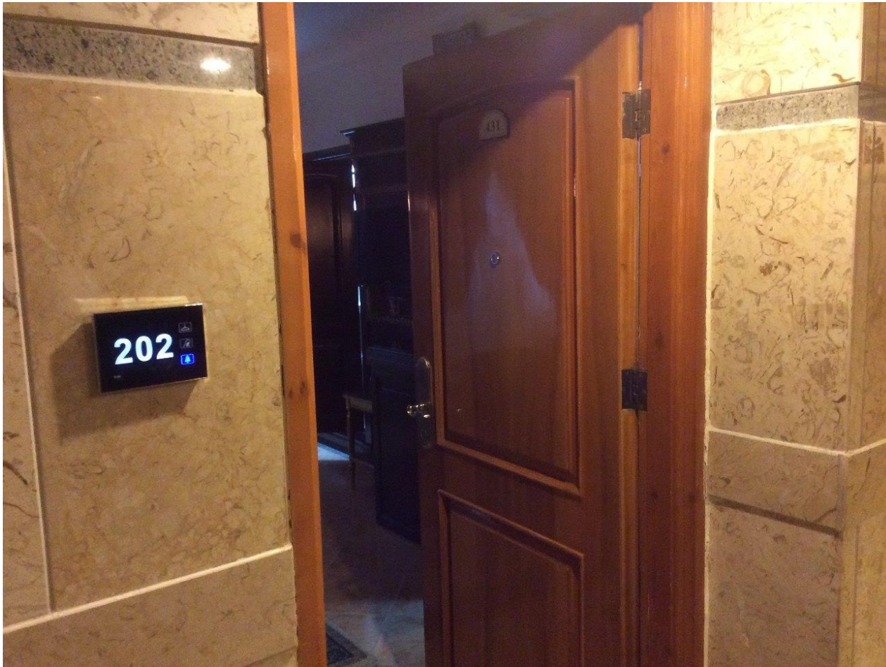
Status panel is installed outside the room, LUNA BELL
